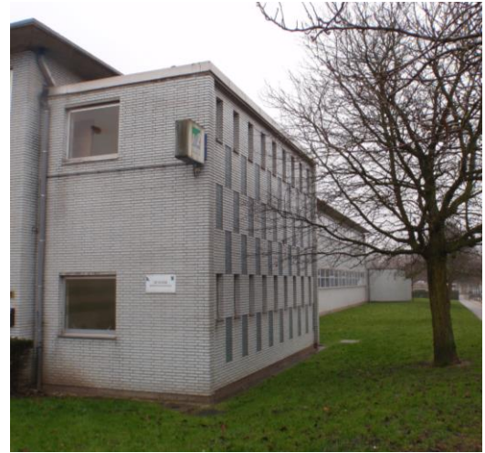
Photo 2 – FACADE P18 SANITAIRES
