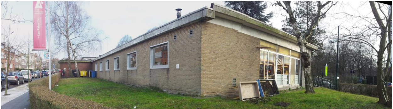
Photo 7 – ECOLE MATERNELLE M3 A DEMOLIR
